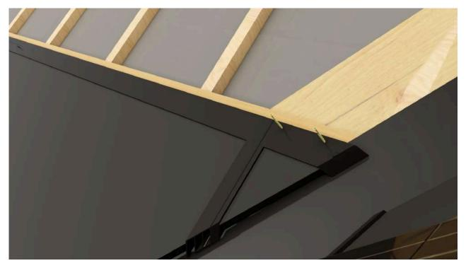
• Add cover flashing to seal the cut section of the dummy panel. Fasten it with self-tapping screws.
