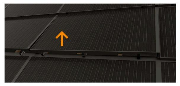
• Once the module has been freed from the clamps, pull it downward. All the cabling and the previous cabling system must be restored to their original state if a new module is being installed.
