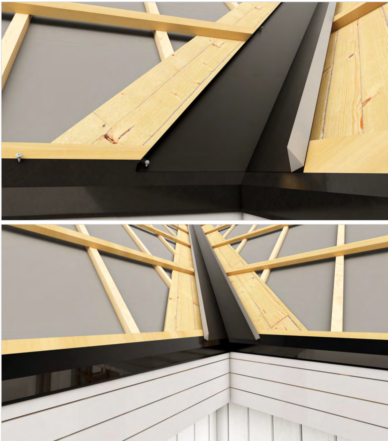
Installation of the valley flashing.
